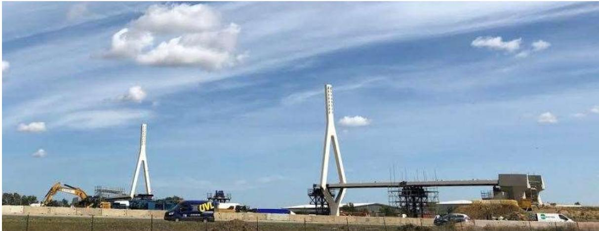
The sections of the deck will rest on the blue temporary supports shown above, while joined to the sections already in place. Eventually the deck will be suspended, as shown in the artist's impression of the finished bridge below.
